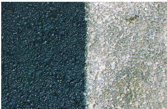
After Seal Coating
